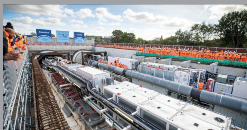
HS2 – Northolt & Euston Tunnels (UK)
